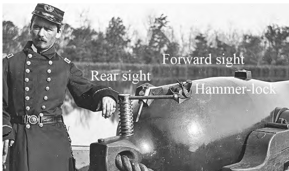
Figure 10: Detail of photograph showing sighting and percussion devices on IX-inch Dahlgren aboard an Union gunboat. (Photo courtesy of the Naval History and Heritage Command)
