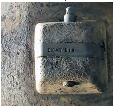
Figure 7: Copper-alloy insert bearing size and serial number in the unused lock of the Dahlgren. (Photo courtesy WLCC)
