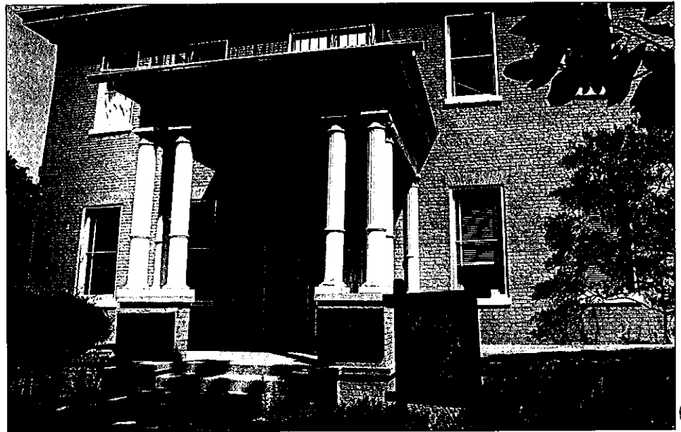
Currently under renovation, Flinn Hall, located behind South Caroliniana Library on the Columbia campus, will be the new home of Women's Studies and African American Studies.
